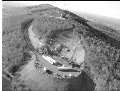
Construction of tower platform at Mars Hill
