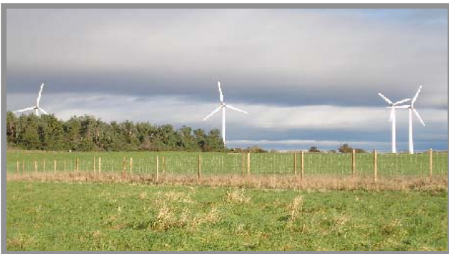
Community wind at Findhorn, Scotland. Four small turbines, max. 150 feet tall, provide 75-100% of the electricity used by the 250 residents and the 4,000 annual tourists.
